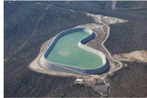
Pumped Hydro (Taum Sauk) 400 MW
