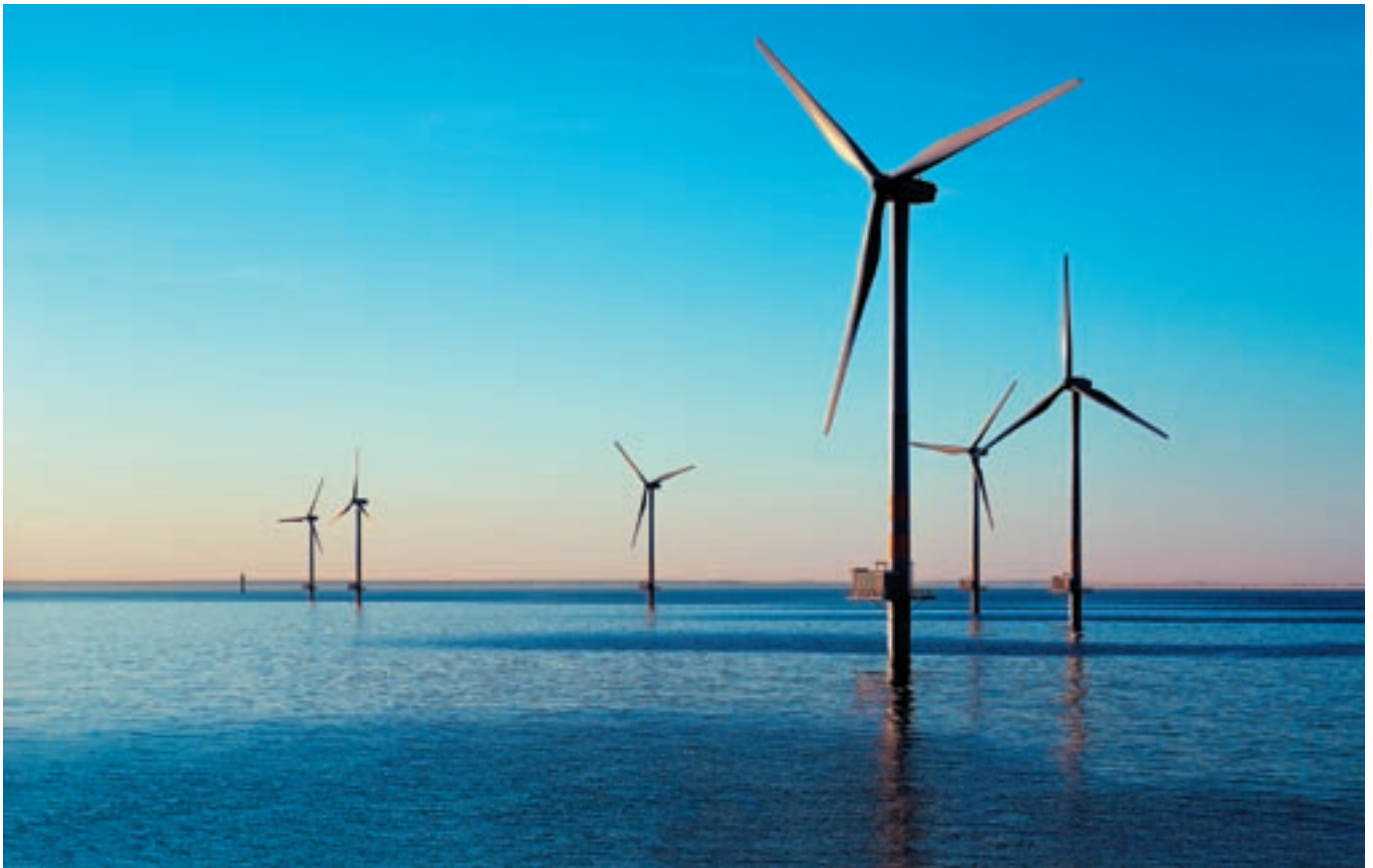
© GE Wind Energy Segment
