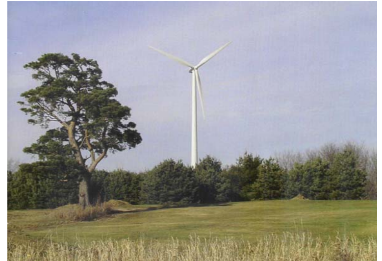
Single 900 kW Wind Turbine Connected to Distribution Line Near Waverly, Iowa
